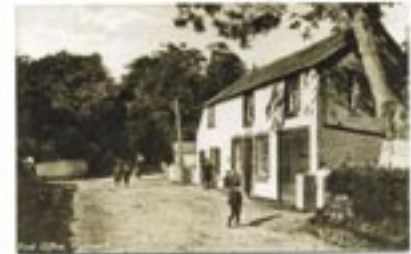
Former Post Office
